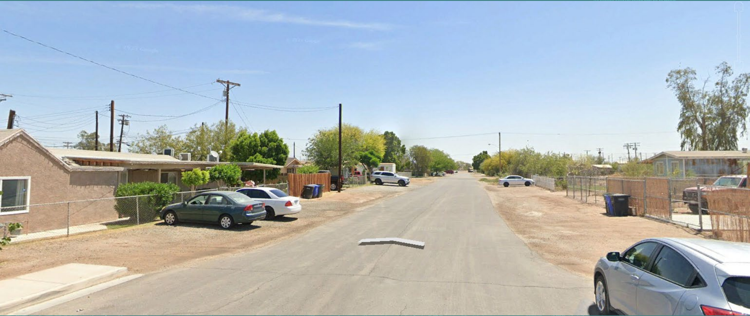
East 7 th Street at Heber Avenue, looking east
