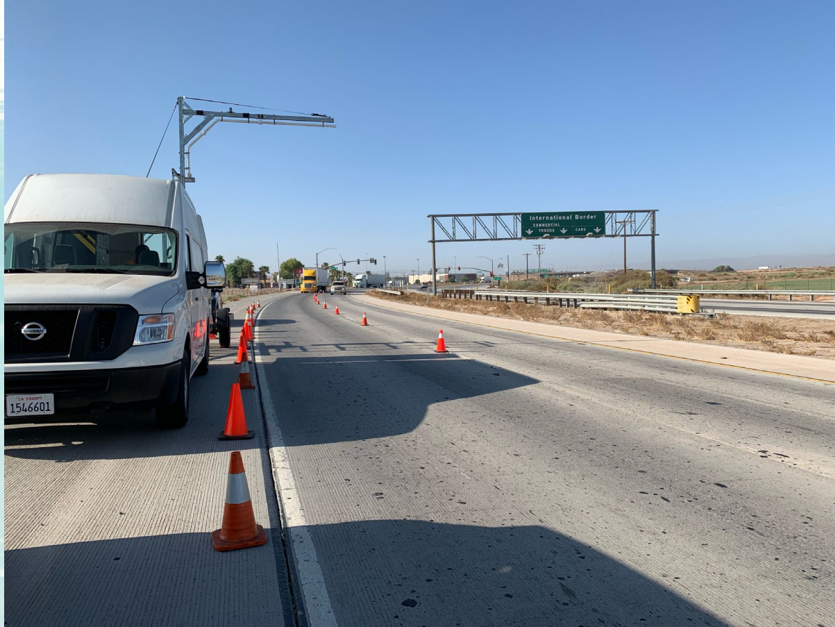
CARB's PEAQS system near the Calexico commercial border crossing
